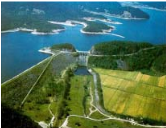
Figure 5 An irrigation reservoir
