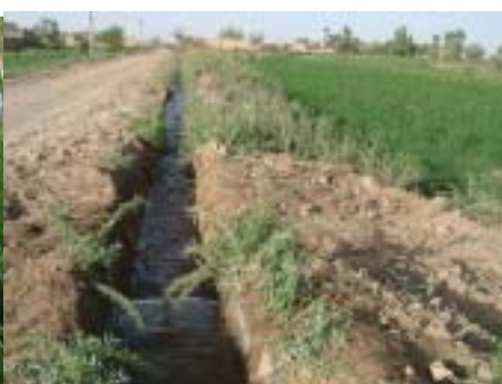
Figure4 Slim flow of canal in Minqin
